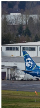
The Alaska Airlines plane maintenance building a MitchellDyer/Associated P
